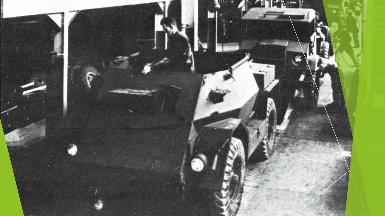
Construction of the armoured hulls was supposed to begin immediately at the NZ Railway Workshops in Petone, but it remains unclear if the order was executed. The chassis, which were still in Canada as late as November 1942, eventually arrived in early 1943, with production starting shortly after. Production ceased by February 1944, by which time 76 vehicles had been completed, 9 were in the process of being fitted with bodies, and 15 chassis remained untouched.
